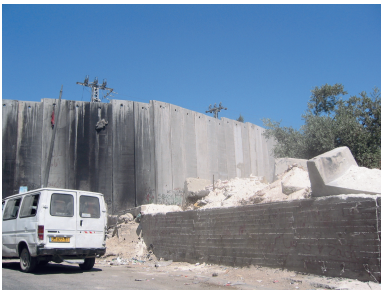
Fig 1. The view of the wall from Al-Quds Medical School (photo: SM Watkins).
