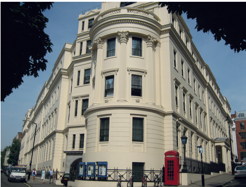
Fig 1. Decimus Burton's original Charing Cross Hospital (1834) (on the right) though the fourth floor and entrance portico were added in the 1880s. Its subsequent expansion can be seen to the left. Copyright © N Black 2007.
